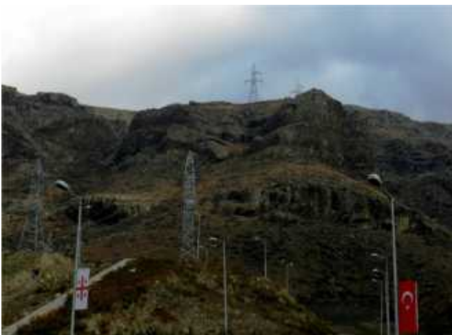
Figure 2. Start point - Paravani HPP substation area
