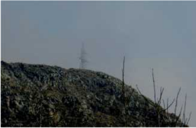
Figure 5. OTL tower in the Paravani section
